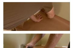
**Consider rolling paper underlay** over the subfloor. It acts as a slight barrier against moisture and makes it easier to slide flooring into place.
