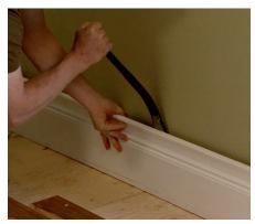
**Remove the baseboards** around the room with a pry bar. Be careful not to damage the boards if you plan to re-install them.
