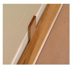
**Place shims** between the first row of hardwood and the wall. Hardwood expands due to moisture, so allow for an expansion gap around the perimeter of the room, equal to the thickness of your plank. If you're using 3/4-inch planks, leave a 3/4-inch gap. These shims must be removed after the installation is complete. The baseboards will cover the gap.
