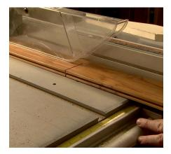
If the planks do not fit exactly across the room, you will need to **cut the first and last rows to equal widths.** If they fit perfectly, you're in luck.
