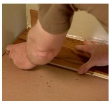
The last few rows of hardwood are often the toughest to install because of the tight space up to the wall. Since the flooring nailer won't fit, use a nail gun or drill pilot holes and use a hammer to nail the last few pieces of hardwood in place. Use a nail punch to help set the nails flush with the surface of the hardwood. Measure and cut the final row of hardwood. And remember to allow for the expansion gap.
