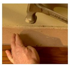
**Slide the last row into place** and use the shims between the final row of hardwood and the wall. Tighten the gap between the final two rows using a pry bar pressed against the shims to protect the walls. Pre-drill holes again through the hardwood and floor. Then nail the final strips into place.
