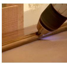
**Drive flooring nails through the tongues of the hardwood** and use a nail punch to set the heads flush with the surface. Repeat the procedure of laying and nailing the hardwood across the floor.
