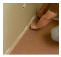
Measure the width of one plank plus the size of the expansion space and mark the paper in several locations along the starting wall. Use the marks you made on the building paper to **snap a straight chalk line.** This is where the tongue edge of the first row of hardwood will be laid. It's important to get the first row straight as it effects the entire installation.
