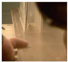
**Cut the first row of hardwood** using a table saw with a sharp rip blade and a rafter angle to protect your hands. Be sure not to cut the tongues off the lengths of the plank.
