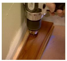
**Align the first strip** along the chalk line, the tongue edge facing into the room, and drill holes every 12 inches, through the hardwood and into the floor. Then drive two-inch ring shank flooring nails through the holes.
